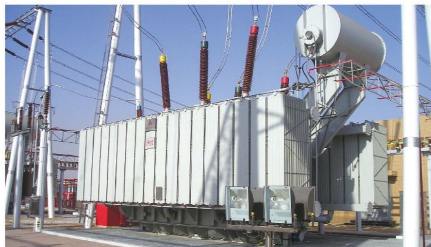
500kV 自耦单相绕组无励磁调压电力变压器 500kV self-coupling single-phase winding voltage regulating power transformer without excitation
